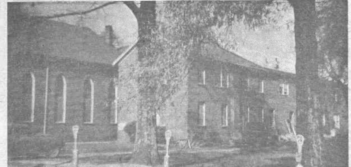
IUKA METHODIST CHURCH was the scene of a cornerstone laying ceremony held Sunday morning, marking the opening of the newly completed addition to the church annex. Rev. G. R. Williams, superintendent of the New Albany district, was on hand to assist the local pastor and congregation of the church. Construction of the new addition was started in September and was completed in January. At present interior painting, cleaning, and redecorating the parsonage is in progress.
